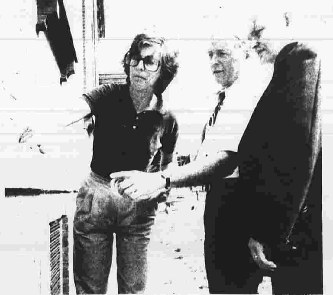
Cheney Hall Inspection Mary McCahon (left), a coordinator for the Connecticut Historical Commission, joins Ed Green of Malmfeldt Associates (center) and Donald Kuoff of the Cheney Hall Foundation to inspect Cheney Hall this morning. Malmfeldt designed the exterior renovations to the hall, which Kuehl said are "more than 99 percent complete," and the historical commission contributed $60,050 to the job. The three checked for any problems in the work, which was handled by the Metro Building Co. Ms. McCahon praised the hall's restoration as an example of cooperation between public and private agencies.
